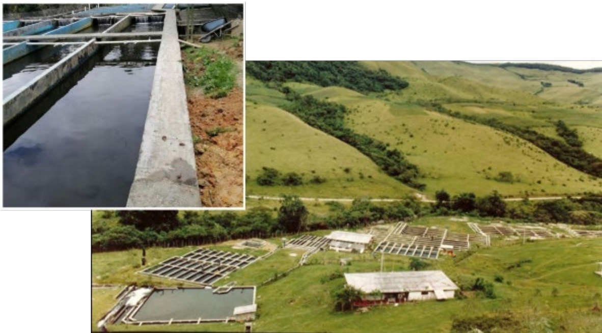
Figure 3: Examples of cement raceways in Colombia. Image reproduced from Roca-Lanao et al. (2020) and http://www.eldiviso.com/ .
