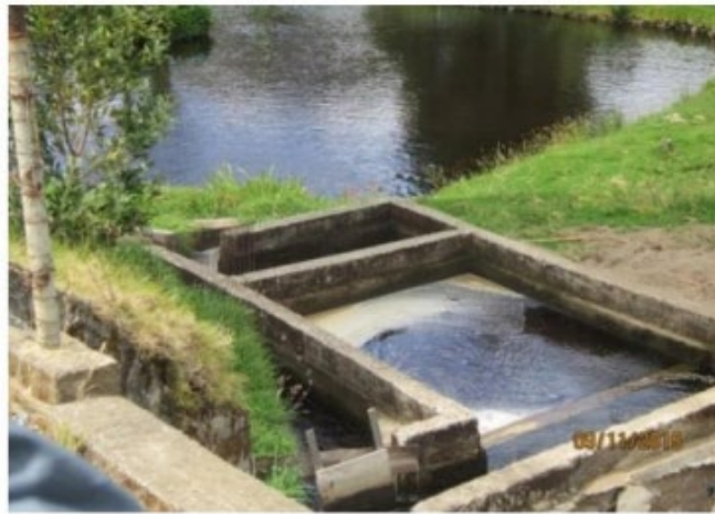
Figure 20: Example of a simple sedimentation filter to collect particulate wastes from a small pond (seen in the background). Image reproduced from Sánchez-Fajardo and Cuello (2015).
