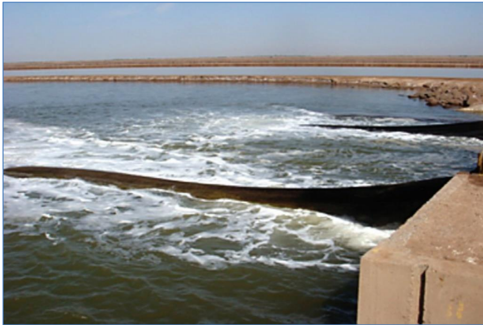
Figure 13. Exclusion infrastructure at canal intakes. From SENASICA (2017).
